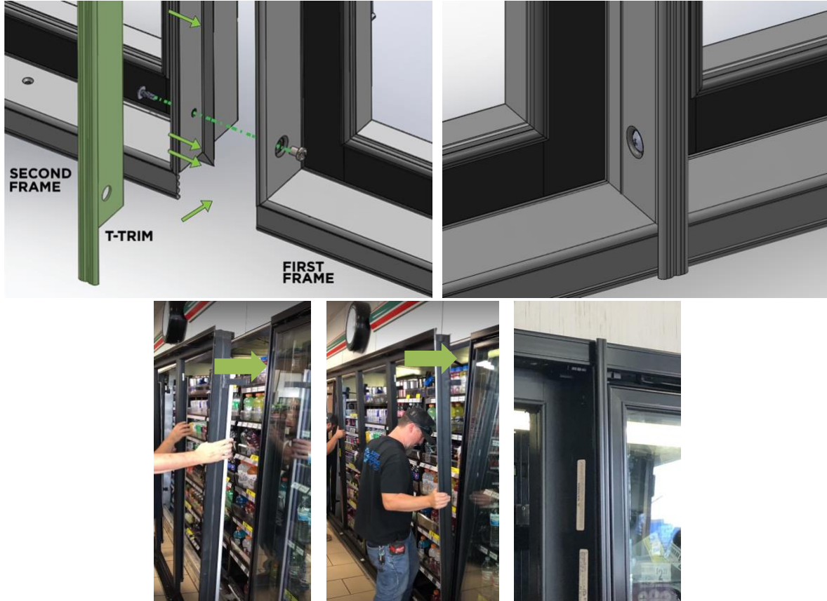
Figure 2.6: T-Trim installation
