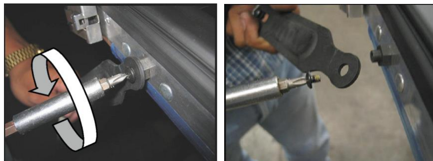
Figure 13.1 Removing hold-open assembly from door.
