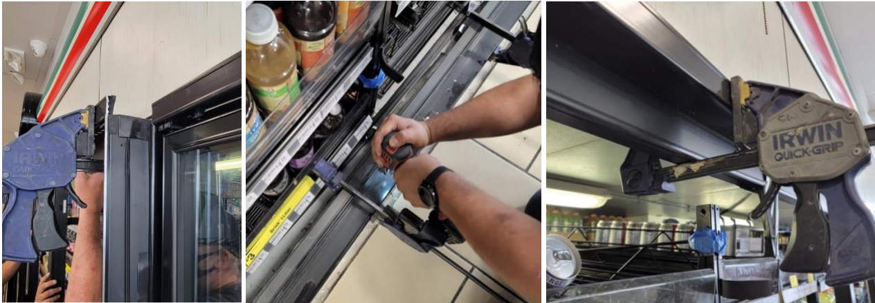
Figure 2.2: Clamps to insert Frame into Net Opening
