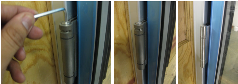
Figure 18.16: Torquing Hinges
