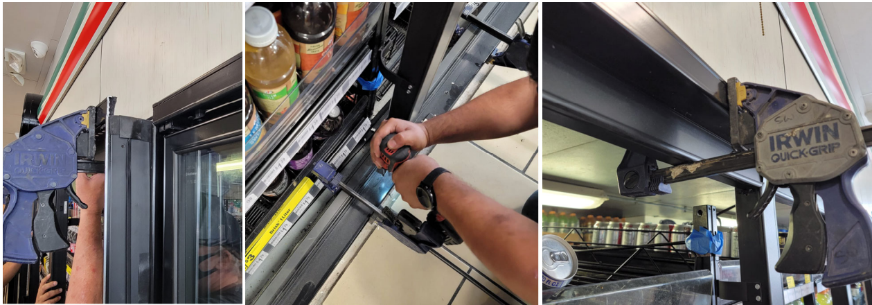
Figure 2.2: Clamps to insert Frame into Net Opening
