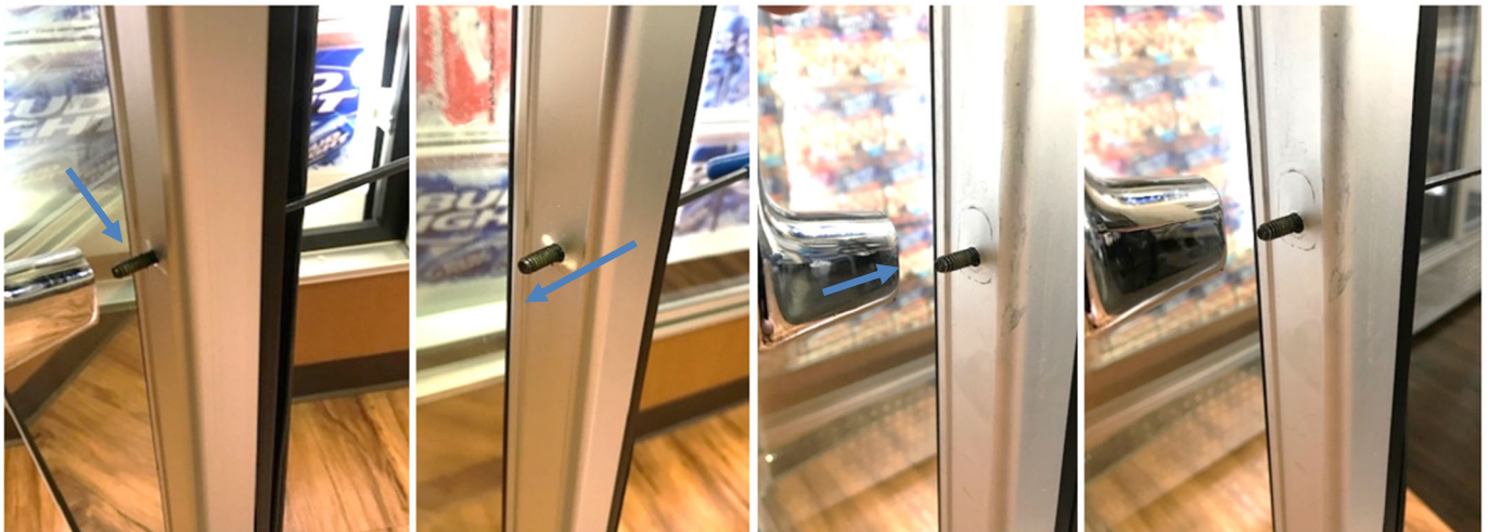
Figure H.2 – Expose screws and secure the new handle
