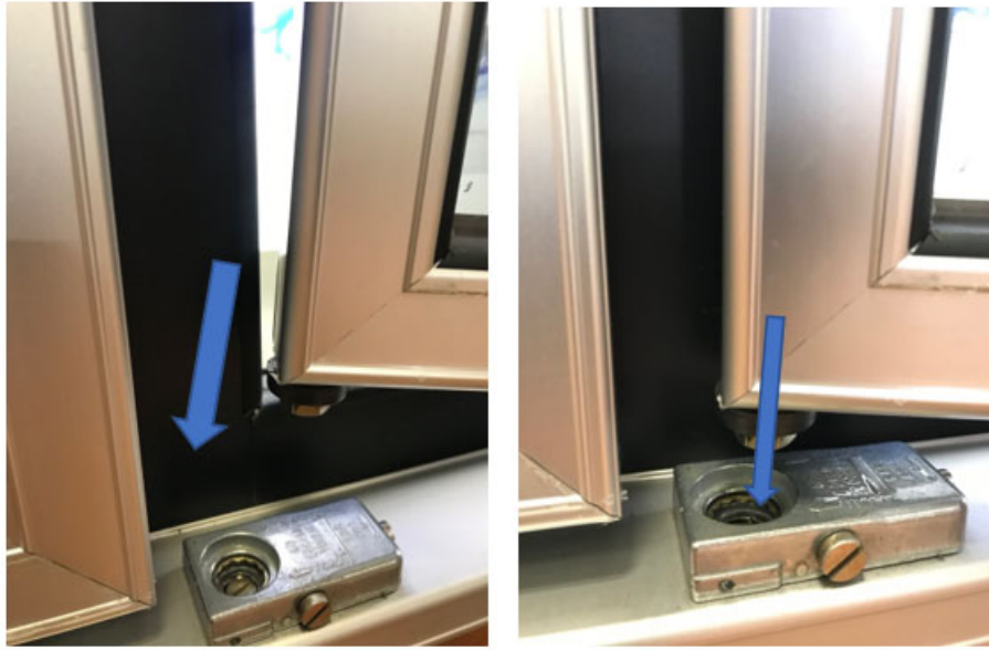
Figure 4.1: Seating Door onto Torque Master
