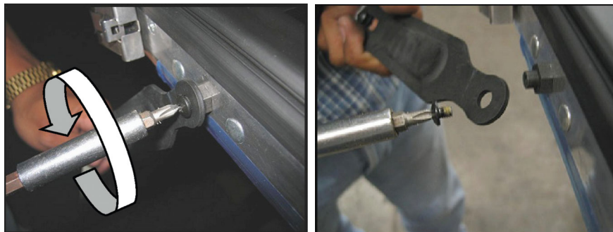
Figure 14.1 Removing hold-open assembly from door.
