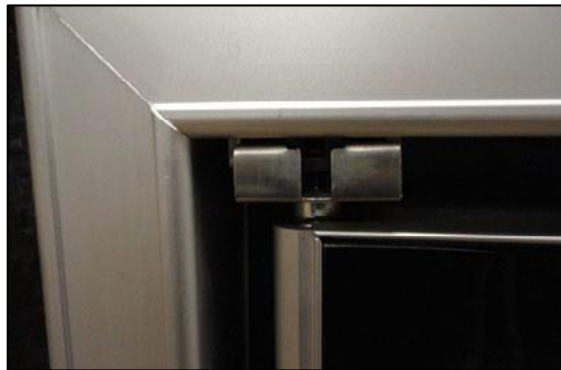
Connect Hinge Pin
