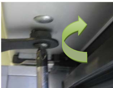
Tighten Hold-Open Screw
