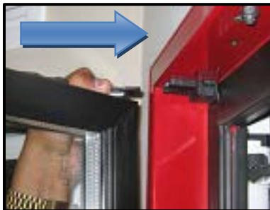
Connect Hinge Pin
