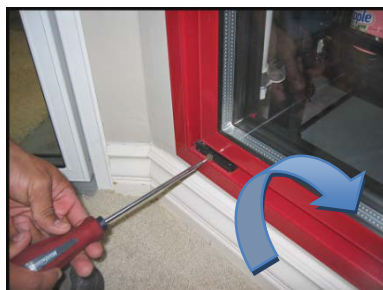
Release TorqueMaster Tension
