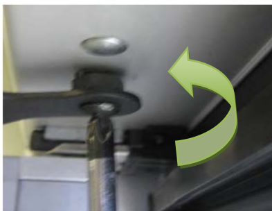
Remove Hold-Open Bolt
