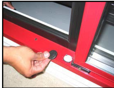
Remove Plug Gap
