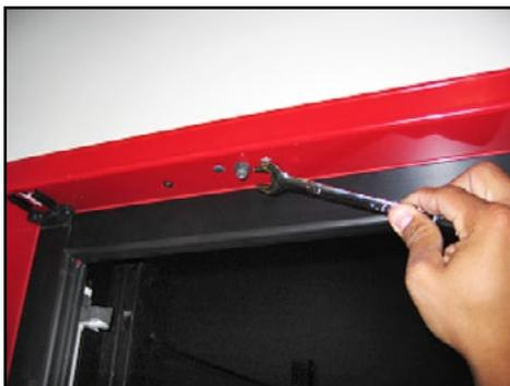
5. Set the door tension swing and correct the door alignment by adjusting the torquemaster (see 'Torquemaster and SAG Adjustment').
