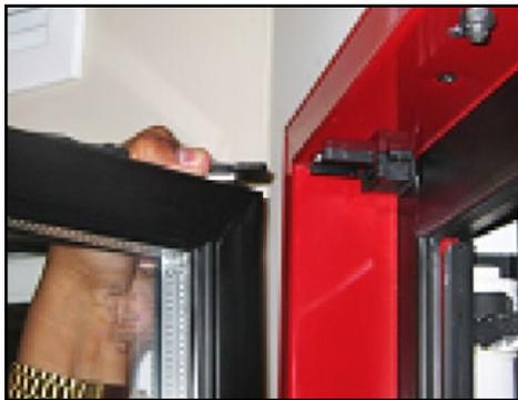
3. Insert the hold-open bolt through the elongated hold-open slot.
