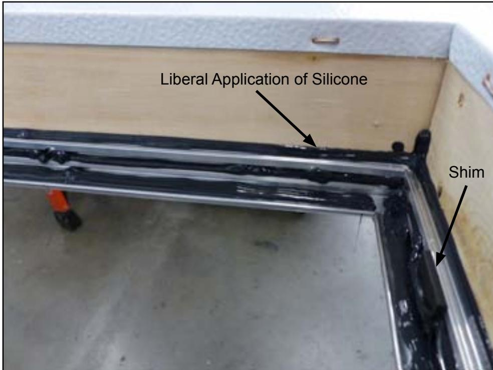
7. Divide the distance between the corners into three equal lengths and mark locations. Apply a liberal amount, several pumps, of silicone Dow Corning 995 at these positions between the edge of the glass unit and the wood frame.
