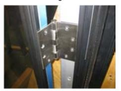
2.2. Next, align either top or bottom spring hinge. Repeat step 1 process and tighten all screw positions on all hinges.
