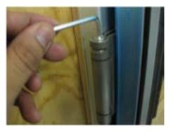
Once at the fourth hole, insert the stopper pin and remove the wrench key.
