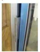
After both pins are in, check the door closing tension. To achieve proper door closing force, move the tension stopper pin from one hole into the next, in either direction, by using the wrench key.
