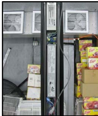
Smart Controller Unit Location
