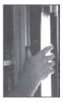
8. Holding lens snugly against top of light fixture, install spring steel clip over lenses. Snap clip into pre-punched holes on each side of mullion. Move to bottom of fixture and install bottom clip.
