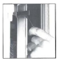
3. Remove ELS lens. Starting at top, pull lens away from front of light fixture that is attached to the frame mullion. If necessary, a small flat-head screwdriver can be inserted between the lens and black mullion plastic, to ease the lens out of the groove. There is no need to remove the lens from the bridge (the black or clear plastic piece connecting the two lenses at the back of the fixture).
