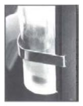
**IMPORTANT:** Bulb insulators must be on each end of bulb before lenses are re-installed. Foam end caps should be securely attached to top and bottom of lamp sockets. (Foam end caps are cut to fit snugly, but if they have become dislodged, or pulled out during changes, they must be replaced!)
